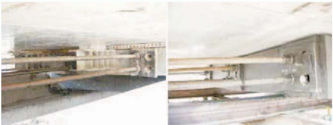
Zambezi River Bridge, incremental launch
